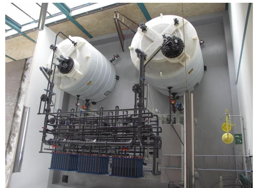
Stationary vanadium flow battery at SYSlab, Risø DTU
